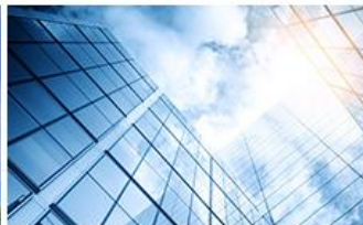
Building exterior wall
